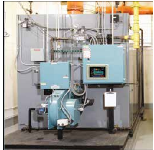
Retrofit your boiler’s dated control system with virtually any boiler or system
