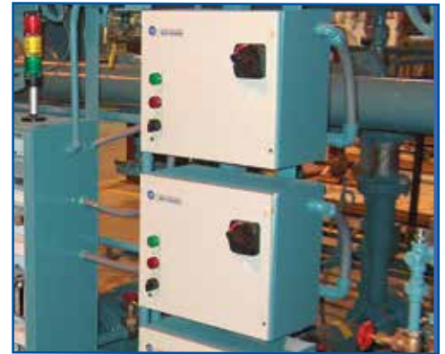
VFD, soft starters, combination starters and contactors available with automatic sequencing and alternation
