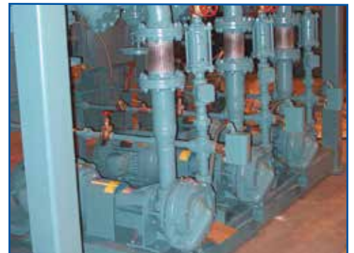
Multiple pump staging
